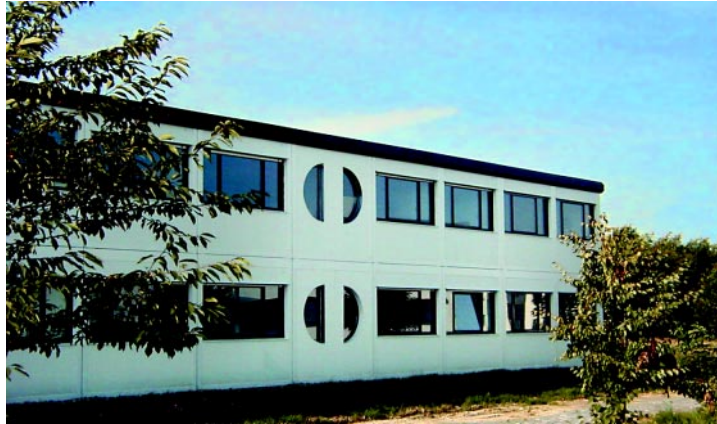
More comfortable offices for dSPACE Paderborn.
