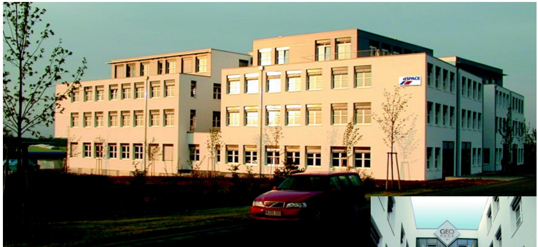
Stuttgart Project Center located at Geopark, Stuttgart.
