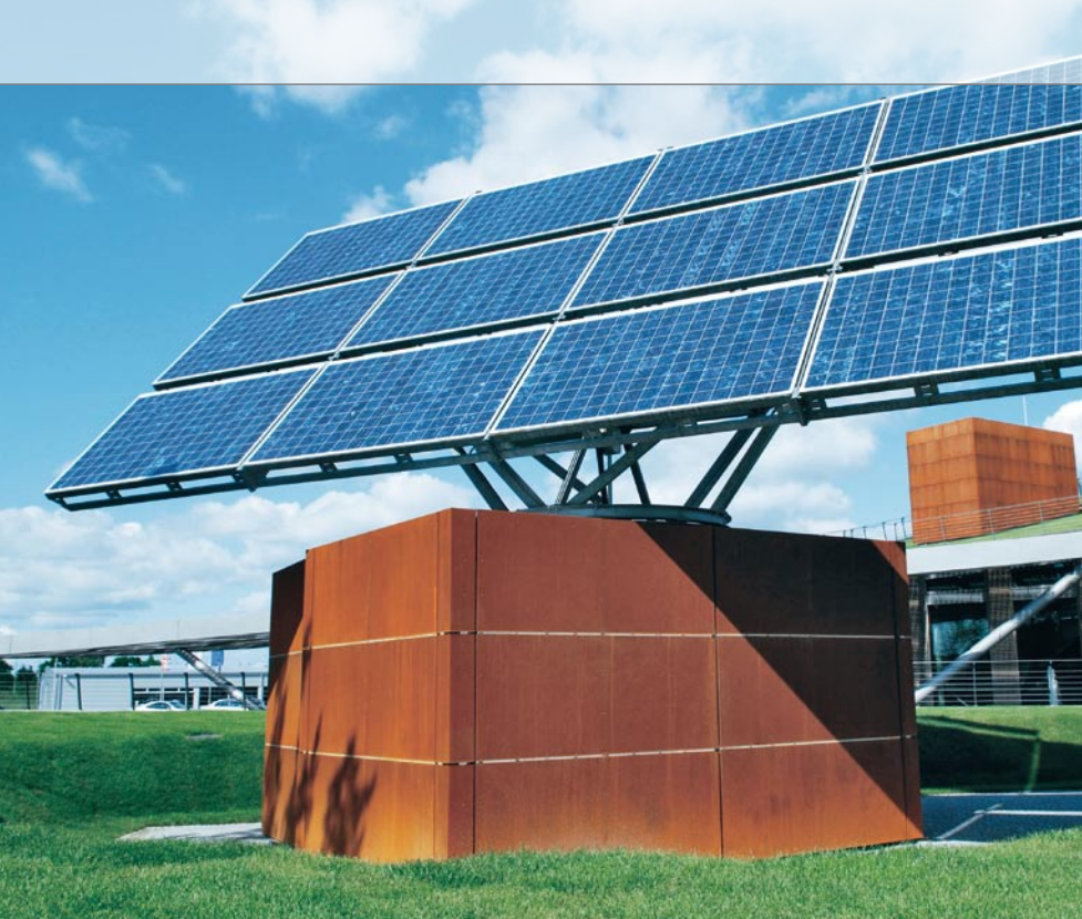
Figure 4: Another Younicos project also uses energy from the sun: This solar power system feeds an autonomous charging station for electric vehicles.
