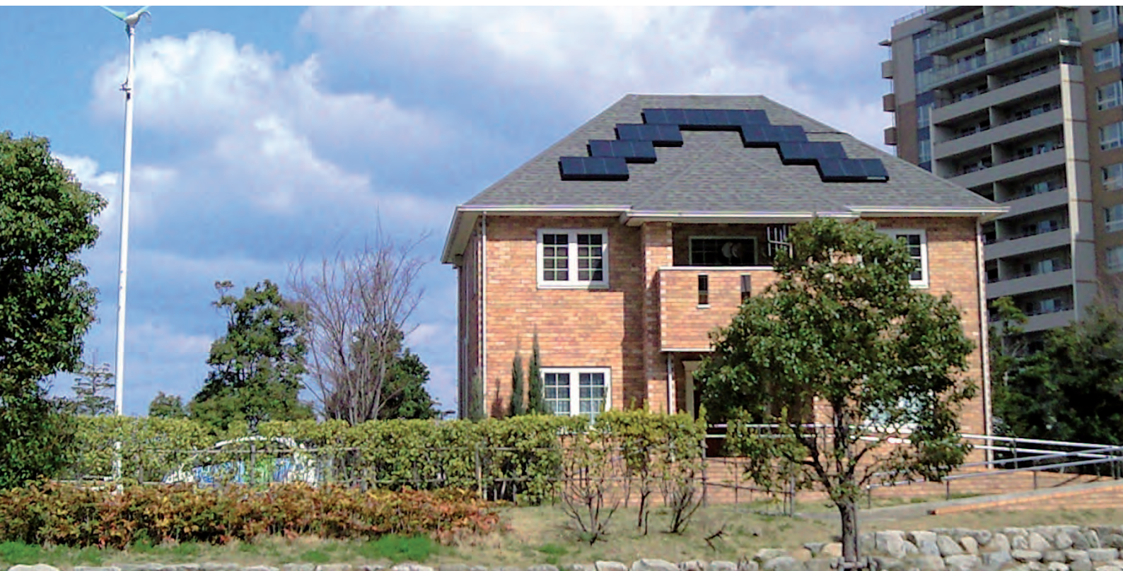
Figure 2: Brick house in Island City in Fukuoka where demonstration experiments are carried out.
