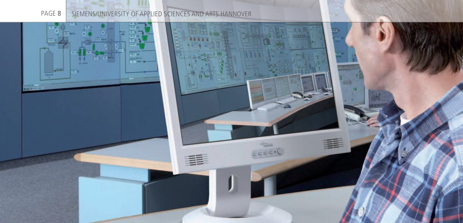
Figure 3: Large steam turbine power plants are automated with the T3000® turbine control system from Siemens AG.
